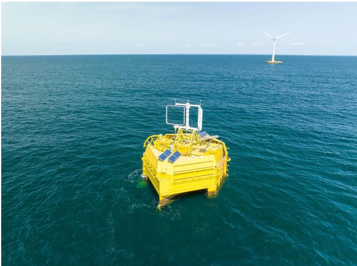
*SeaLhyfe 1-MW offshore electrolyser, operational since Q2 2023<sup>13</sup>.*
