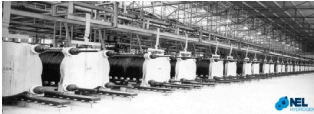
A 135MW alkaline electrolyser facility in Norway, operational from 1953.
