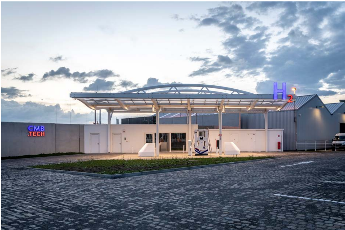
CMB.Tech fixed multi-modal gaseous hydrogen bunkering facility.
