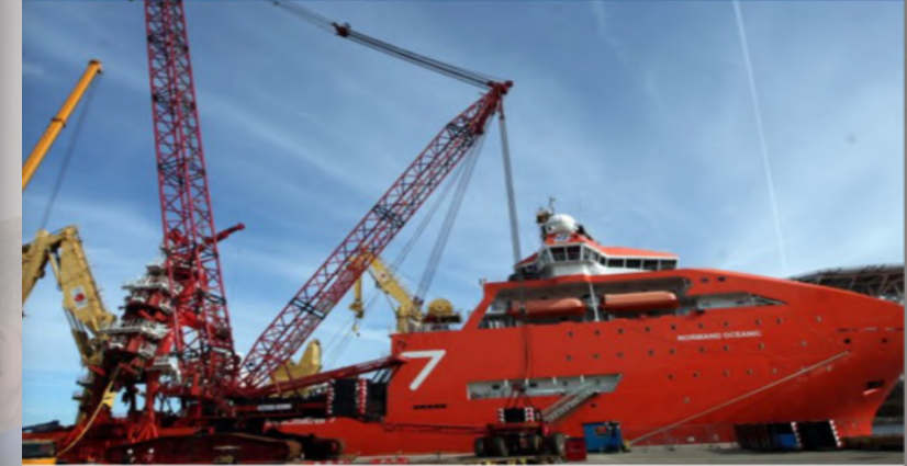
MJR Deliver Design & Construction of Electrical Power Distribution for Back Deck Equipment Spread
