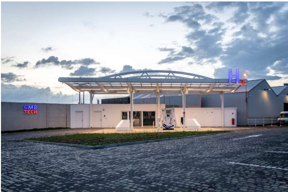
CMB.Tech fixed multi-modal gaseous hydrogen bunkering facility.
