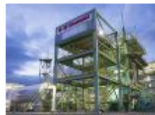
Hydrogen Liquefaction Plant
